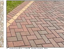
Concrete unit pavers to match existing
