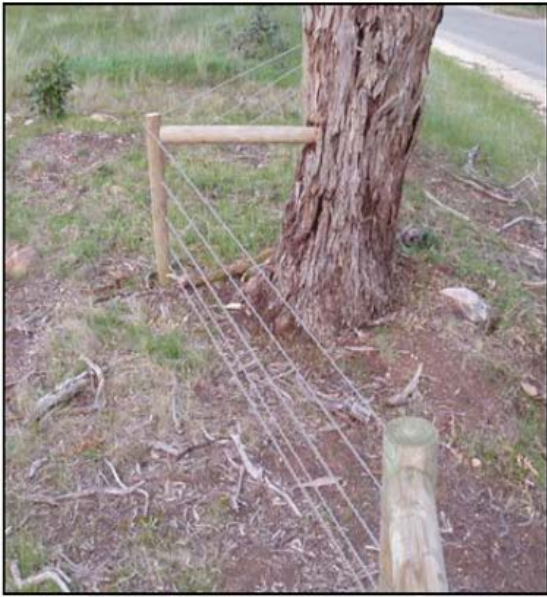
Image: A simple strut arrangement that allows a fence to deviate a short distance around a tree. Wires are not attached directly to the tree, thus minimising potential damage to the tree.
