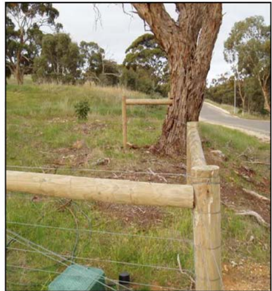
Image: A simple strut arrangement that allows a fence to deviate a short distance around a tree. Wires are not attached directly to the tree, thus minimising potential damage to the tree.
