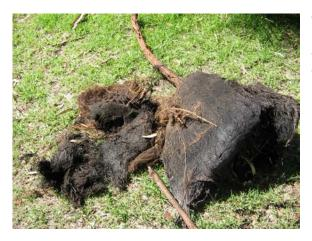
This is a picture of tree roots that had grown in a pump chamber and actually prevented the pump from working. This caused the effluent to back up from the septic tank and into the house.
