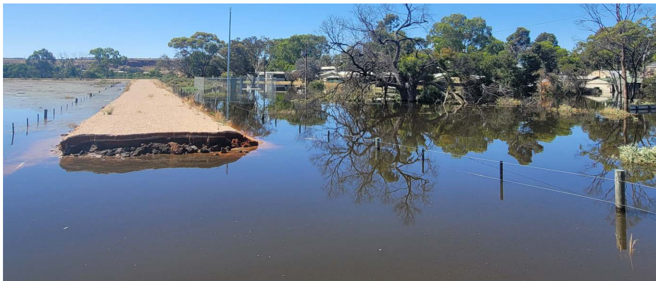
Levee breach at Cowirra
